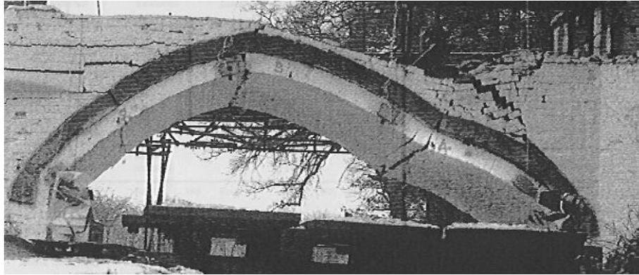
Fig. 7. The Prestwood bridge: the collapse mechanism.
