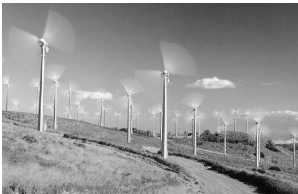
Figura 1.5: campo eolico montagne Theachapi, California.
